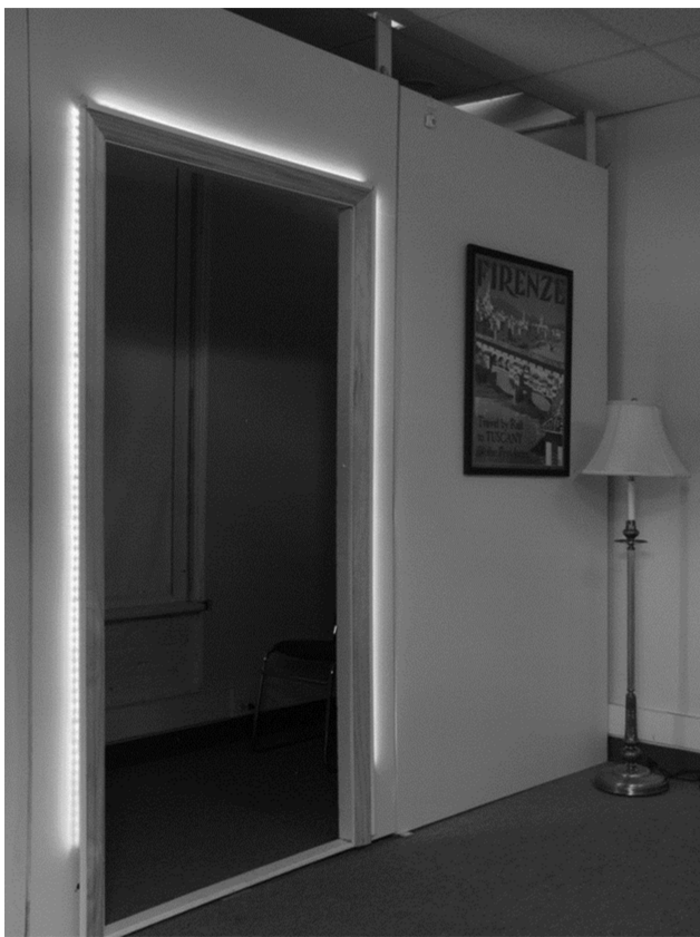
Figure 2. Amber LED lights to outline the bathroom door. Credit: Dennis Guyon, Lighting Research Center, Rensselaer Polytechnic Institute.
